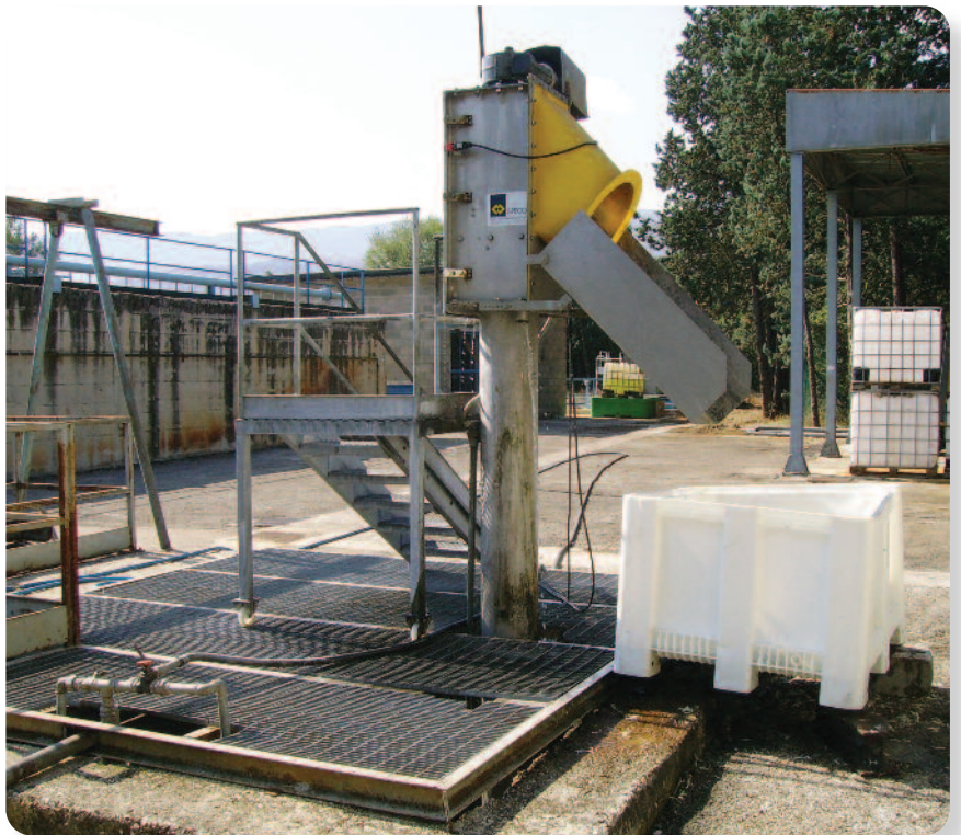
Open Channel Installation
