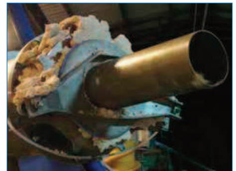
Tapioca processing (SEPCOM Industrial Vertical)
