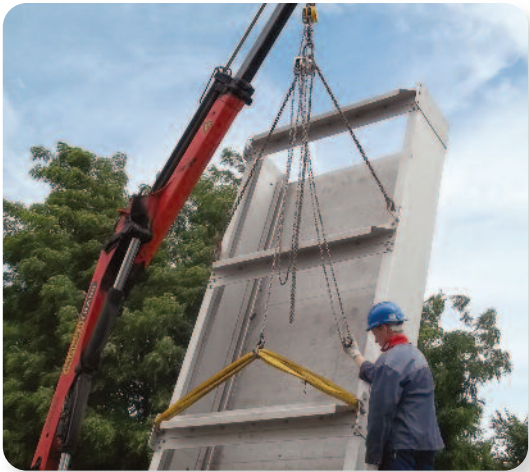
The next section is moved into place.
