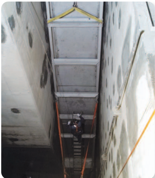
Final assembly and inspection of 180 foot screen.
